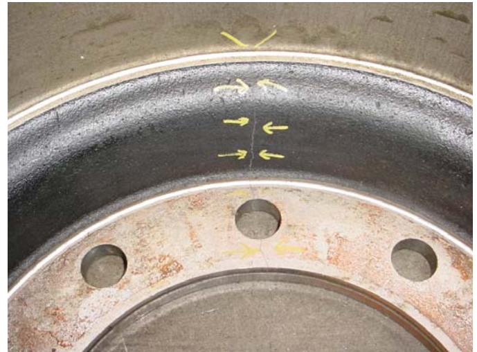
Example of drum cracking.
